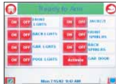
Lighting and Appliance Control
